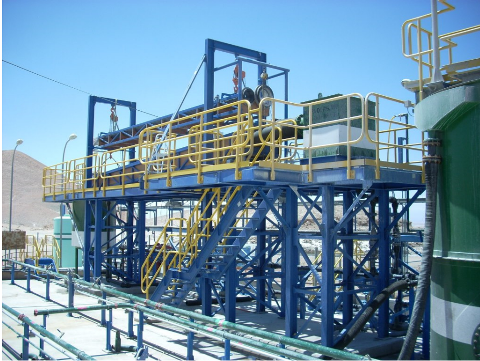
Figure 1. Photograph of the experimental open channel flume used at Chuquicamata, Chile
